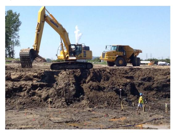
Photo 1. Excavation of existing materials from confined disposal facility.
