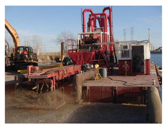
Figure 6. Broadcast capping system<sup>™</sup> placing residual sand cover.
