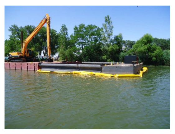
Photo 2: Mechanical dredge removing TSCA sediment within silt curtain containment.
